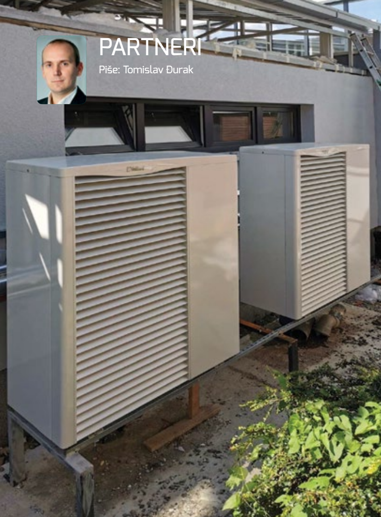
Dizalice topline aroTHERM VWL 155/2
