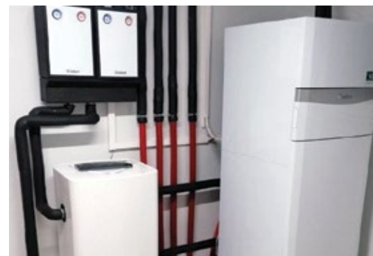
aroTHERM split (ispod) i uniTOWER (iznad), Cesar's
